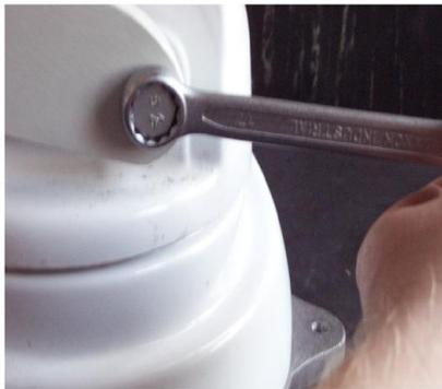
7. Lift up the dish, retighten 1 bolt to keep the dish upright.
